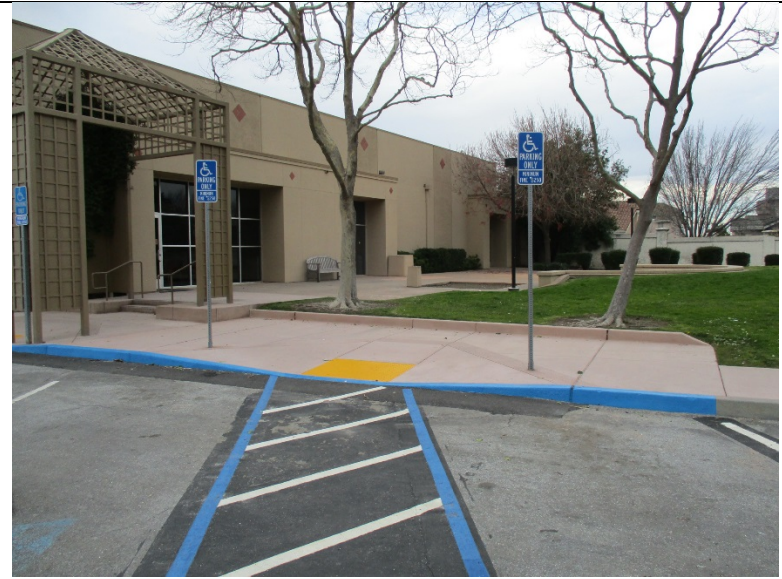
NEW CURB RAMP AND SIGNAGE AT THE MARINA COMMUNITY CENTER
