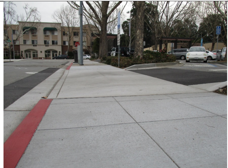
NEW ACCESSIBLE DRIVEWAY APPROACH AT TOLER AVENUE PARKING LOT
